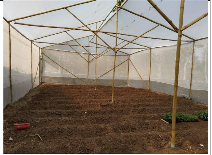
Figure 8. 12: Completed Bamboo polyhouse structure from Balapur village
