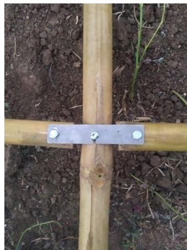
Figure 8. 5: joinery of bottom ties and central column
