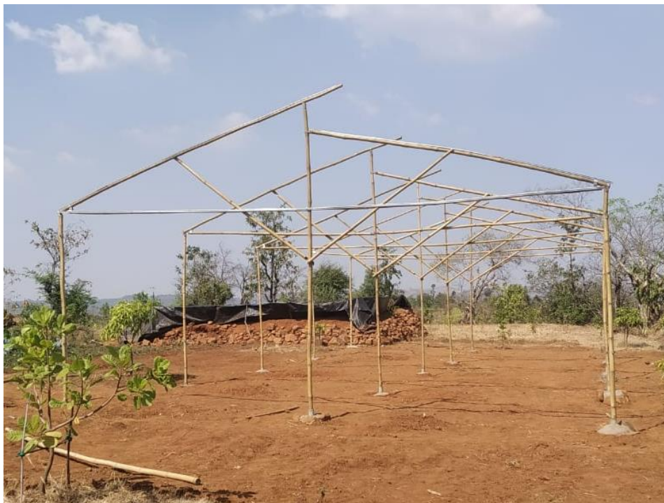
Figure 8. 9: Erected frames of the polyhouse (Image from Ramkhind site)
