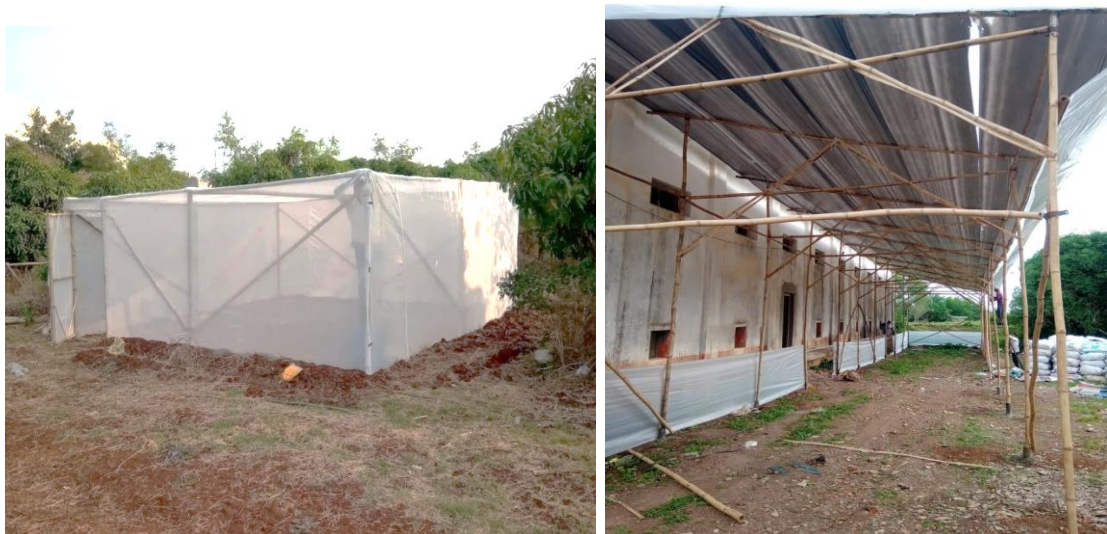
Figure 6. 3: Bamboo structures visited during the field visit a. Structure used for protected cultivation experiments, b. a structure used as an industrial shed
