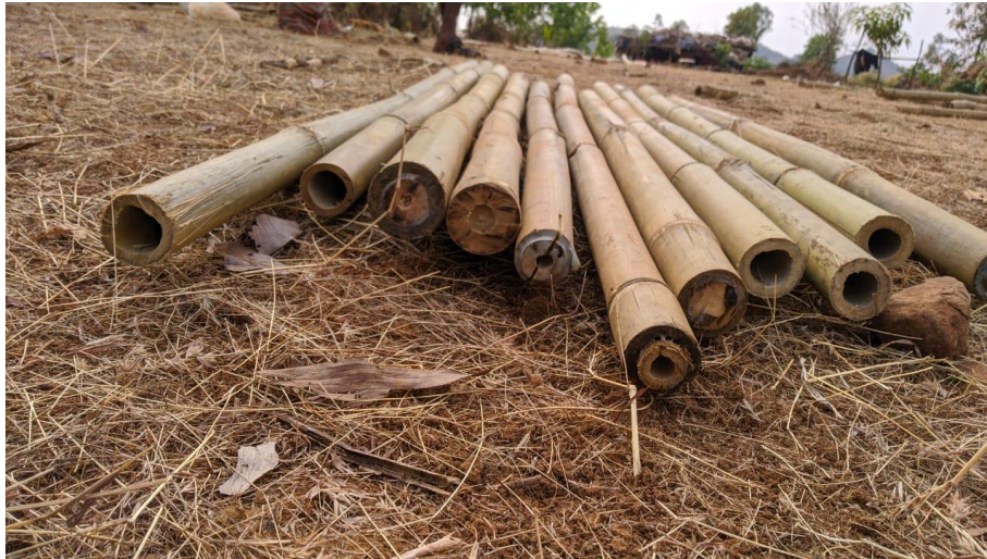
Figure 8. 8: Bamboo inserts for strengthening the joint
