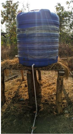
Figure 8. 13: Elevated Tank for drip
