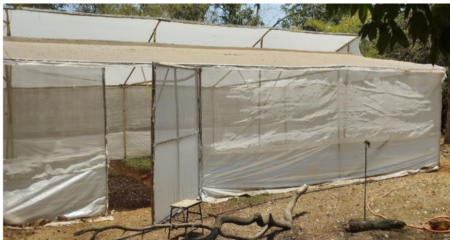
Fig 1: Polyhouse using Conventional Shed-Net
